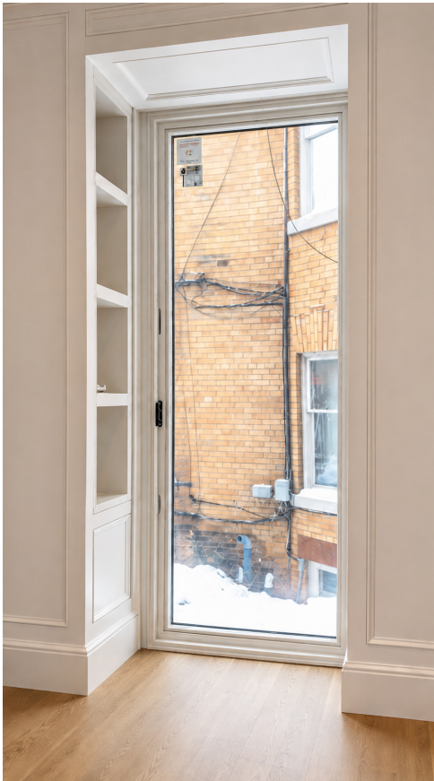
Side-mounted operation shown in a finished-floor casement condition.
